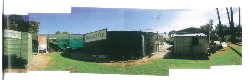
05 — Rainwater tanks, shade houses and community gardens work together in an integrated hydraulic system to recycle and reuse water. Photo taken in 2022.
